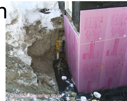
Building Science Corp.
